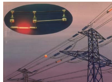
Paris Airport, FRANCE. Working since 1973!
